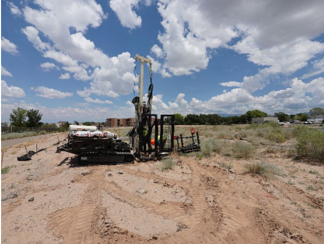
Photo 13: View of auger drilling at borehole B-7 at the subject property.
