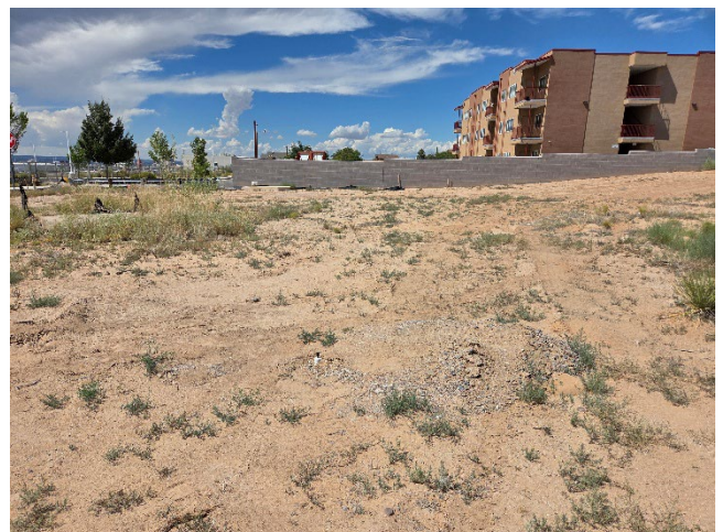
Photo 24: View of LFG-9 capped between monitoring events at the subject property.
