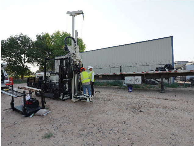
Photo 1: View of dual tube borehole sampling at the subject property on June 30, 2025.
